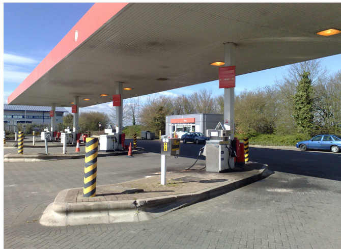
Ashford's Diesel Station Due for refurbishment during 2008
